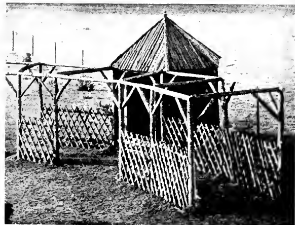
SUMMER-HOUSE AND PERGOLA AS ERECTED IN THE REV. H. E. HODSON'S GARDEN. (See page 382.)
