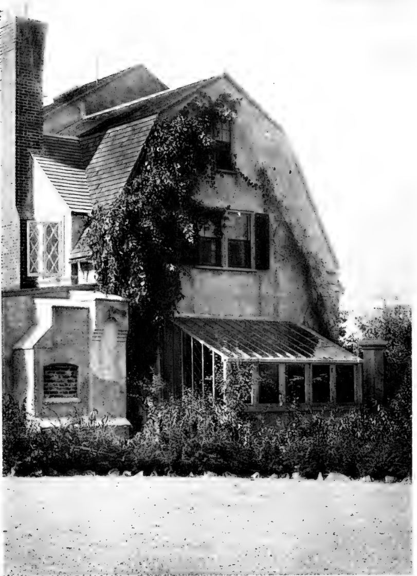
A lean-to type of greenhouse, such as has been built on the east wall of this house, is within reach of almost any owner of a small country place
