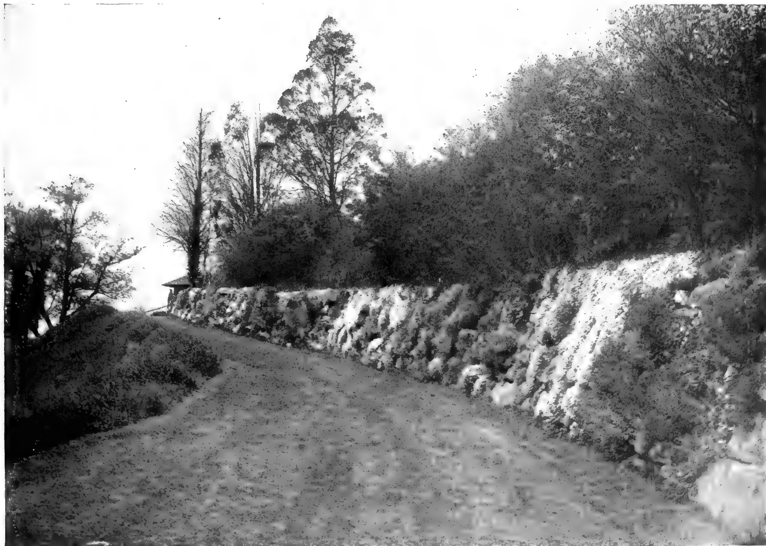
The new attractive way of treating a retaining wall. Build it with ample soil pockets and plant rockery-plants in the interstices
