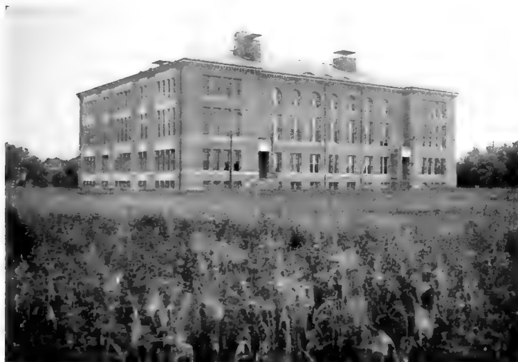
Fig. 2. Before planting, showing what violence every large new building, no matter how good, does to the landscape until trees, vines and shrubs are planted in such a way as to connect architecture and nature
