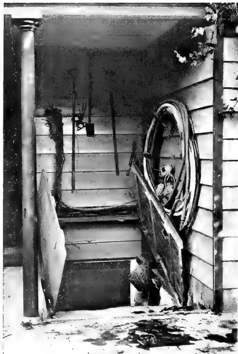
The unpromising proposition we started with. The cellar door and a bit of the porch
