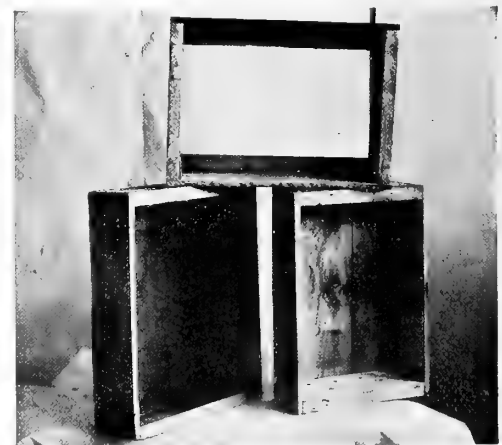
233. The top box with the zinc bottom holds the sand, the middle one the water pan, and the bottom one the heater
