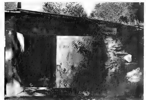
201. A cheap, efficient fruit storage cellar. Two sides are against a bank of soil; air spaces are in the walls. Good ventilation and dryness are necessary
