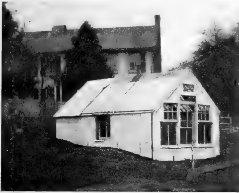
This little 10 x 16 greenhouse cost $41 for materials, including heating apparatus. The section at the rear is a tool shed
