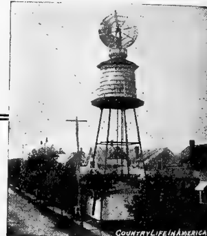
Erected for Shawomet Water Co., Shawomet Beach, R. I.
