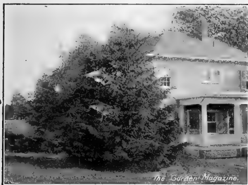
Screen to gardener's cottage. Moved 1905.
