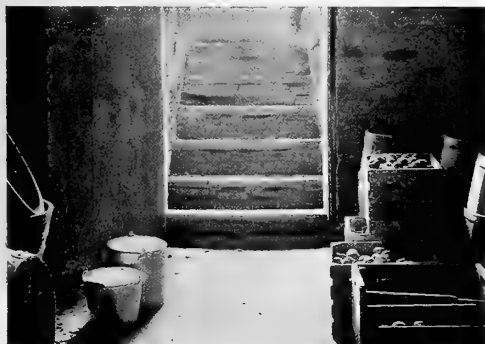
199. A typical home cellar with earth floor. When properly ventilated and dry, it will keep fruit as well as more expensive storage cellars
