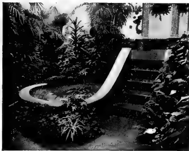
Interior of Concrete Greenhouse
