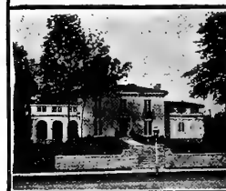
KELSEY HEATED HOUSE at Pelham Manor, N. Y. OSWALD C. HERING, Architect New York City
