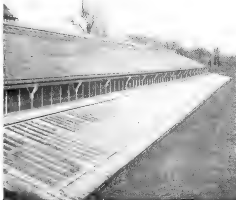
Permanent coldframes of brick and cement. If frames are wanted next to greenhouse, provision must be made against snow falling on frames
