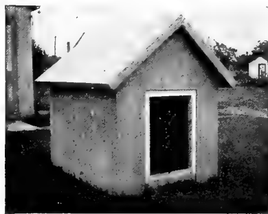
Concrete Dog House
