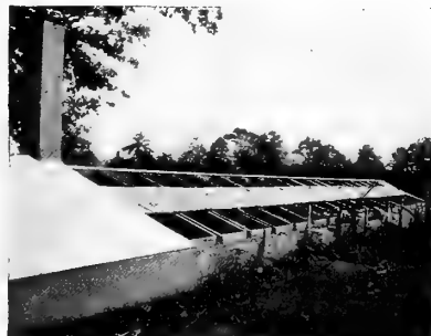
A Concrete Greenhouse During Construction
