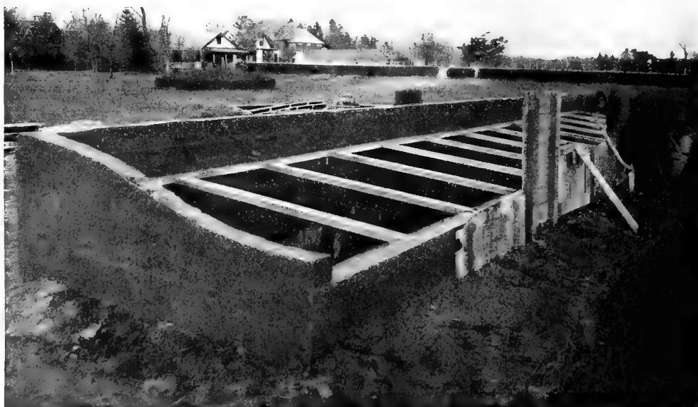
A concrete frame for a hotbed will last a lifetime; wood soon decays. Note the high back protection for the frames
