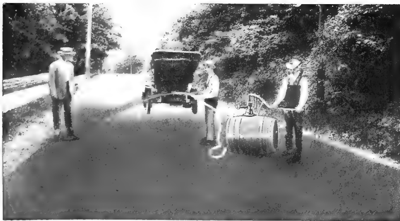
One barrel of Asphaltolene will oil 100 to 140 square yards of roadway. Two men can oil 2100 to 2910 square yards per day with our oil pump and sprayer.
