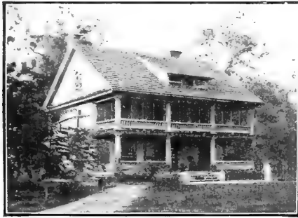
Residence of S. E. Wing, Mechanicsburg, O. E. E. Holman, Architect, Philadelphia, Pa.
