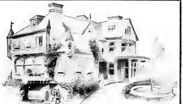
Showing pump in cellar connected with pneumatic pressure tank
