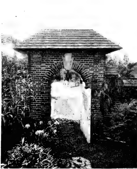
The simple masonry arch and wall, effectively framing the vista beyond
