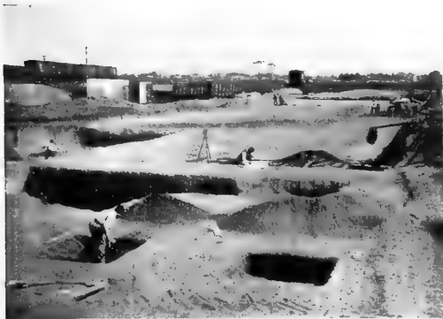
Starting the foundations at Garden City
