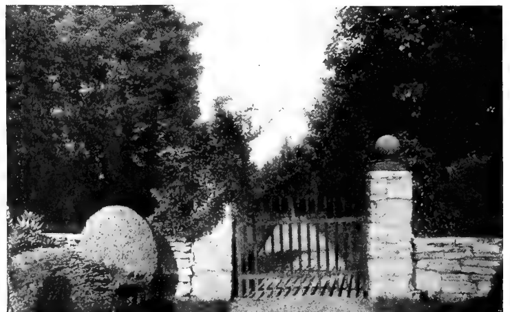
The stone piers are the feature here and harmonize with the lines of the avenue beyond
