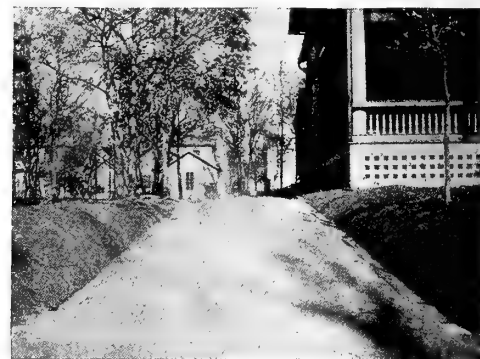
Make your driveways of cinders instead of concrete and have them last longer
