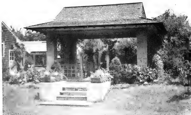
The formal summer-house combined with steps. Effective for small open lawns, giving a positive viewpoint
