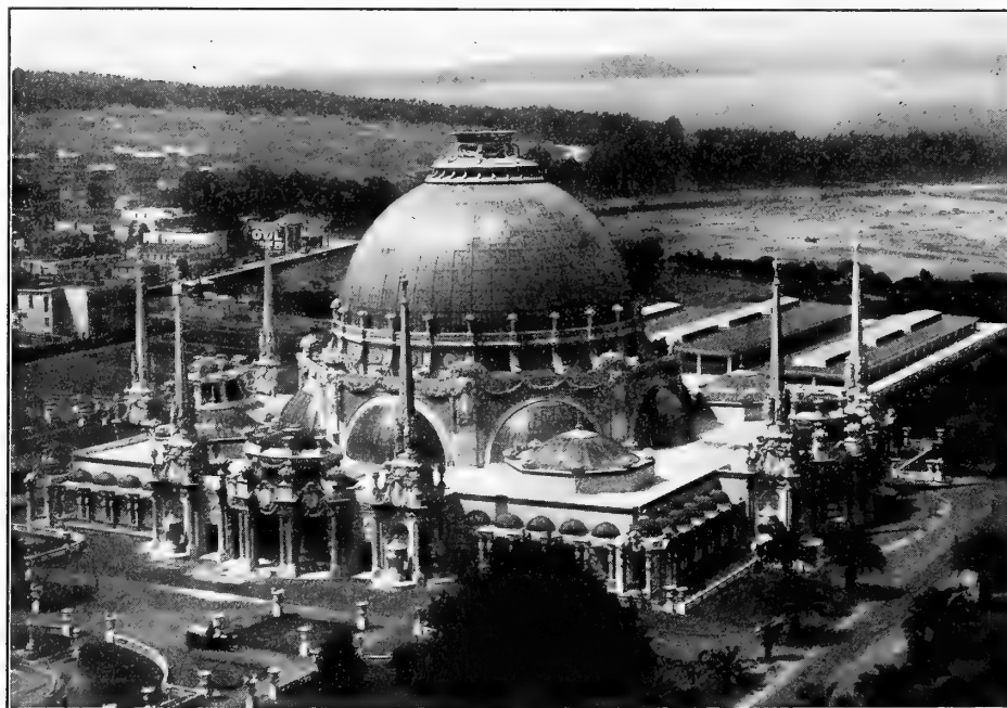
The Palace of Horticulture, taken at a point 125 feet above the ground. The building is 600 feet long and 300 wide. The dome in the centre is 186 feet high and 152 feet in diameter. The architecture of the domes and minarets resembles that of the mosque of Sultan Ahmed I. at Constantinople, while the details of the facades, spires and other decorations reproduce the eighteenth century French Renaissance
