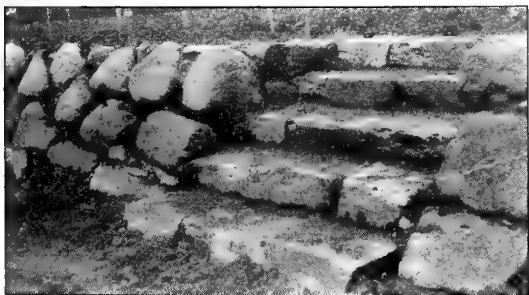
Just built The small plants are already set in the crevices
