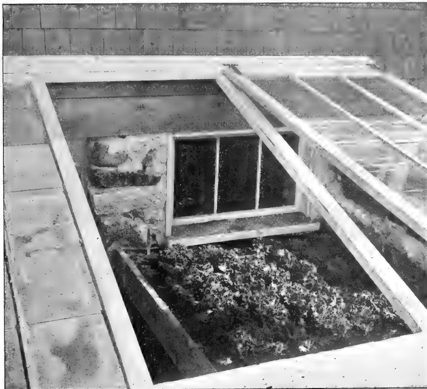
This 4 x 4 ft. bench in a sash covered leanto with door opening into the cellar will furnish enough lettuce for the average home table
