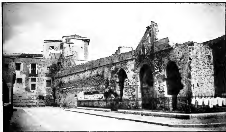
INSIDE THE MONTALTO BASTION.
