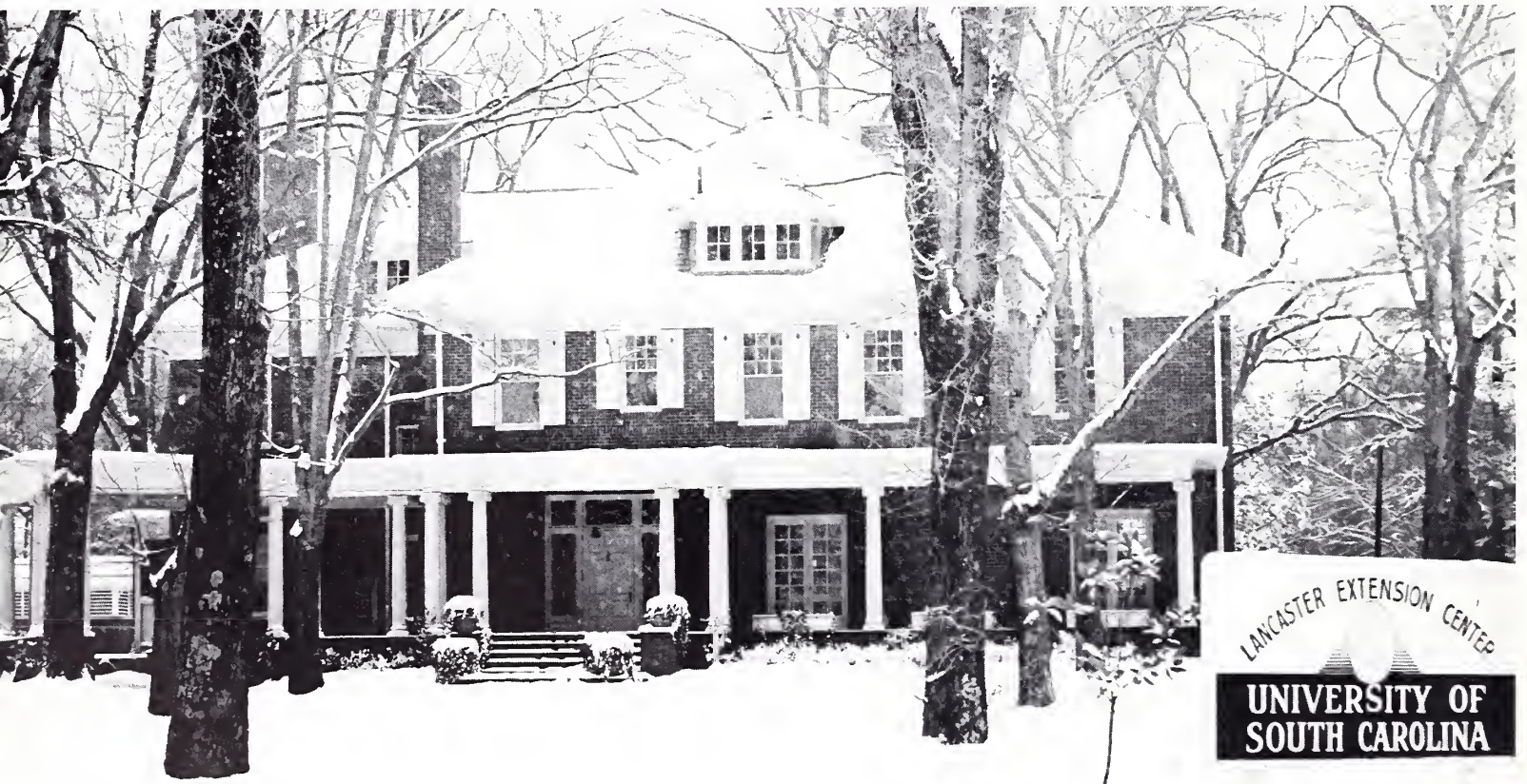
The Main Building of the Lancaster Center.
