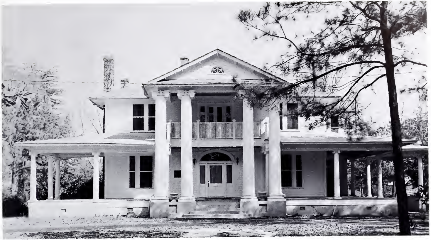
Wallace Hall, Florence Center Student Activities Building.
