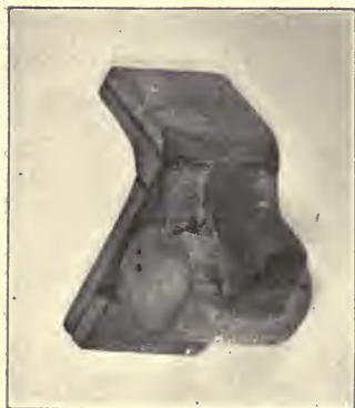
FIG. 34.—VALVE ROD BEARING PATTERN.
