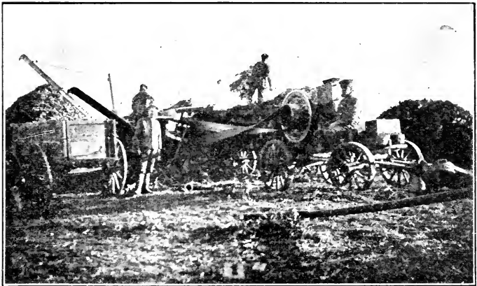
FIG. 105.—Driving With Long, Heavy Belt, Showing Sag.
