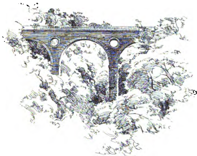
The Pease Bridge.
