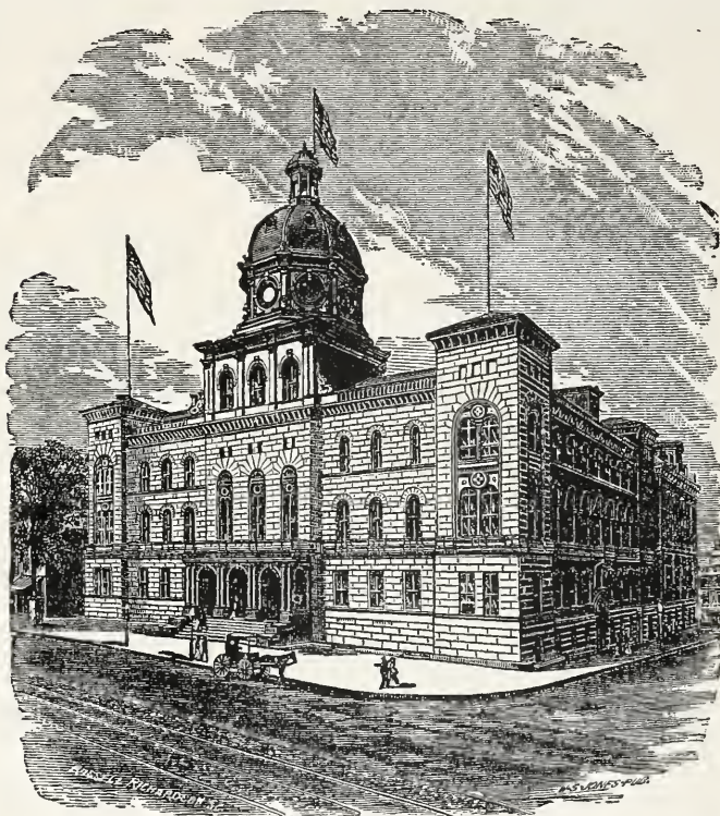
CITY HALL, PORTLAND.
