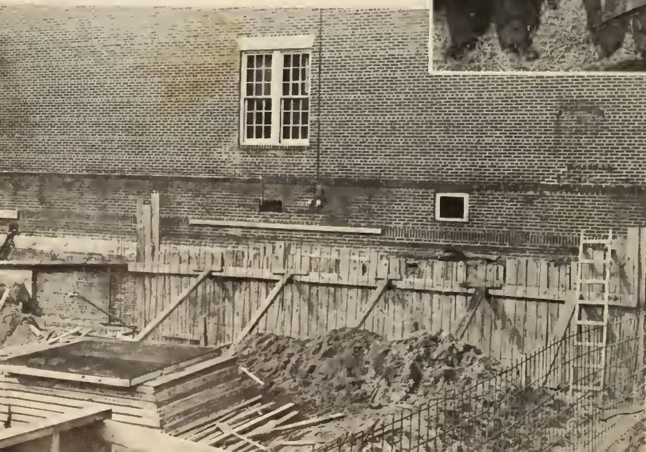
FOUNDATION UNDER WAY
