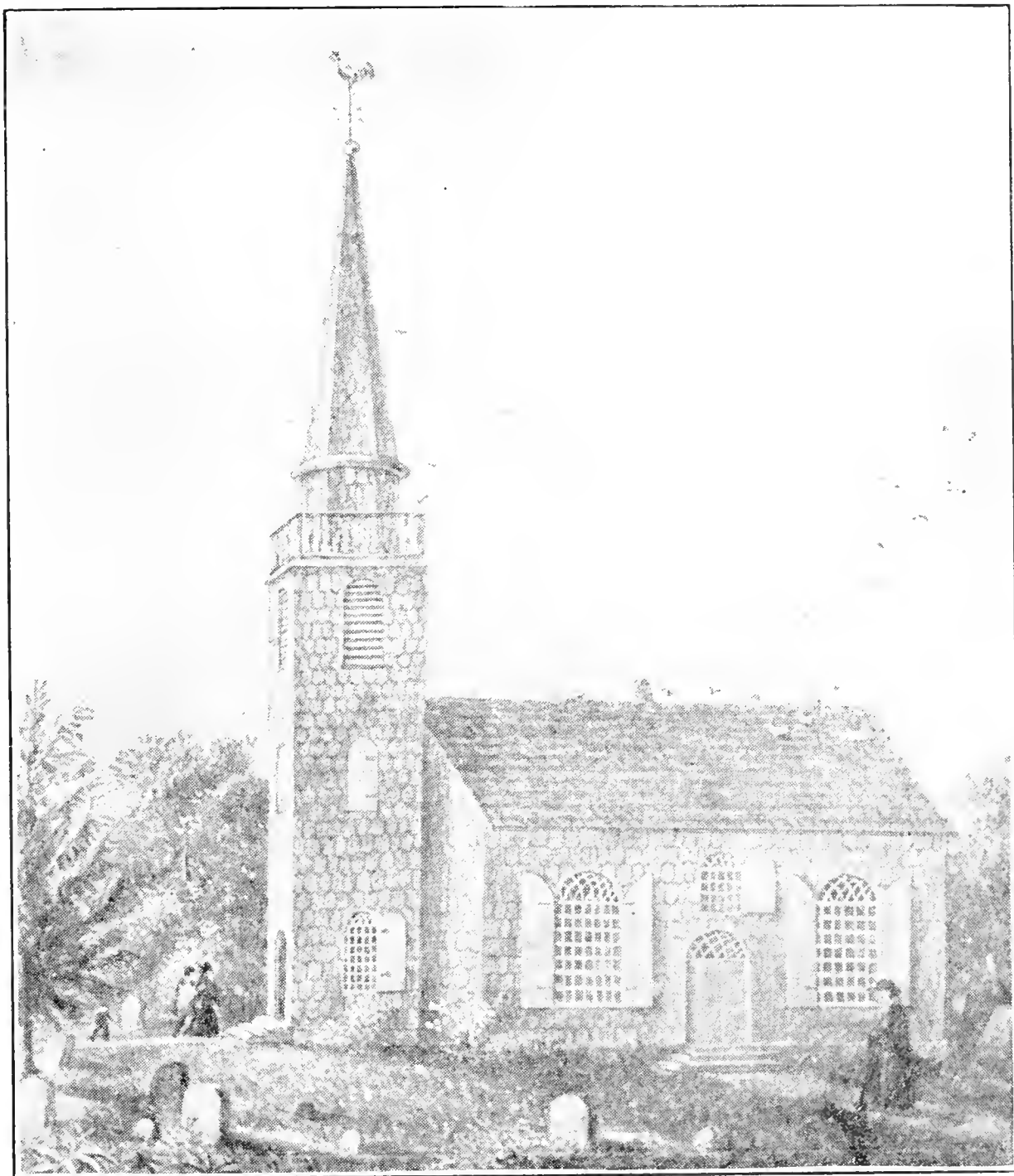
St. George's Church, Hempstead, L. I. Rebuilt 1822.
