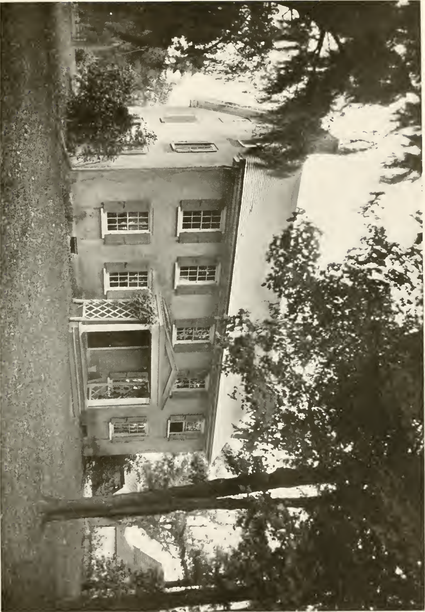
EDWARD FRENCH HOUSE, NEAR WEST MOORESTOWN, N. J., 1770 As remodeled, about 1850, to face the Camden Turnpike
