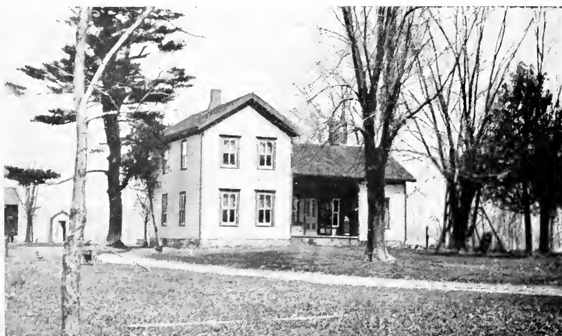
RESIDENCE OF ISAAC WEBB MARTIN. BUILT IN 1856.
