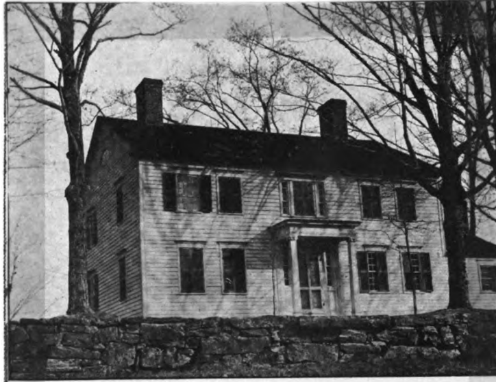
House built in 1807 by Jeremiah Fuller on site of Capt. Abraham Fuller's house, and on or near site of Dea. Joseph Fuller's house of 1738--40, Kent, Ct.
