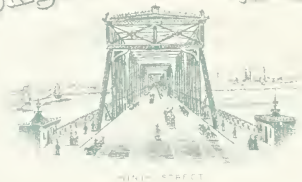
Ninth Street Bridge--the first four track bridge across the Allegheny River. Built by the Pleasant Valley Railway Co. to accommodate the Electric Street Cars.
