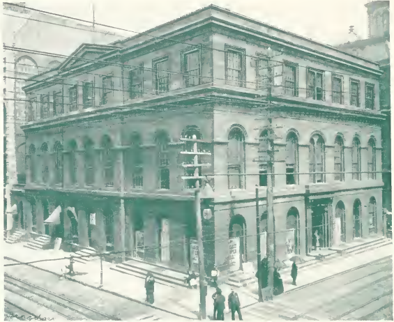
The old Post Office, corner Fifth Ave. and Smithfield St., which was the terminus of the Pleasant Valley Street Railway at the time that it was changed from Horse Cars to an Electric Line.
