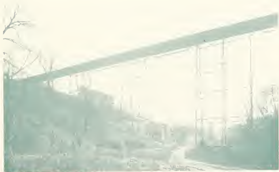
Jacks Run Bridge (or High Bridge) connecting Allegheny and Bellevue. This bridge is six feet higher than the Brooklyn Bridge at New York. Built to accommodate the electric cars of the Pleasant Valley Street Railway Co.
