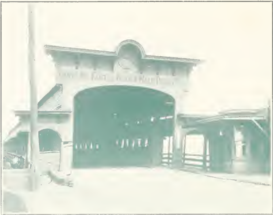
The old Ninth (or Hand) Street Bridge which was replaced by the new steel four track bridge to accommodate the electric street cars of the Pleasant Valley Line.
