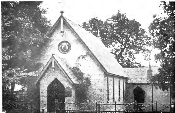
Trinity Episcopal Chapel, Excelsior, Minnetonka Lake, Minnesota, of which I took an active part in building, about 1863.
