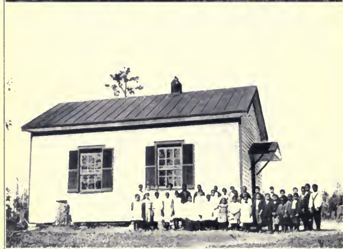
Poplar Lawn School, Va., "Before and After."
