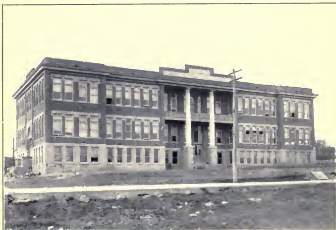
New District Graded and High School, Princeton, W. Va.
