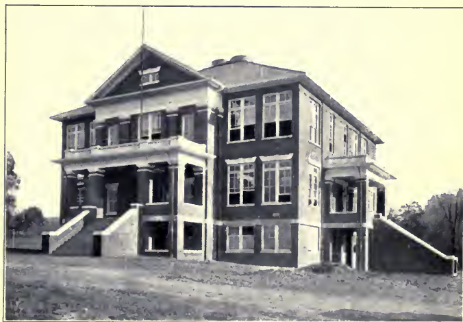
Young High School, Knox County, used as a model for rural high schools now building in Tennessee.
