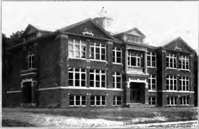
District High School, Clendeik, Kanawha County, W. Va. New building.
