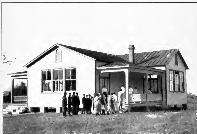
New school, three rooms, Burkeville, Va.
