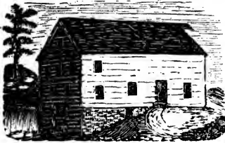
Old Mill at Hibernia.
