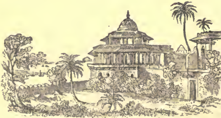
Fortified Palace at Allahabad, Hindoostan.
