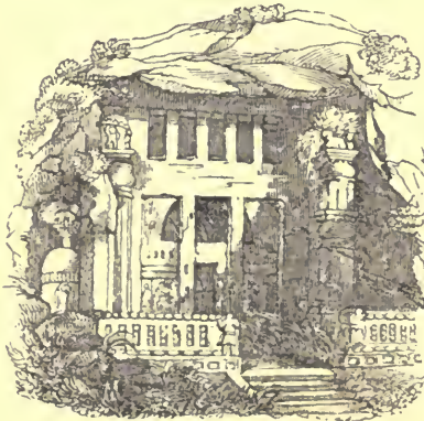
Excavated Mountain of Kenneri.
