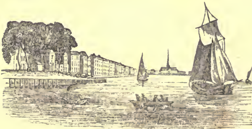
View of part of Rotterdam. 2 E
