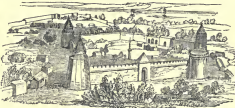
Castle of the Seven Towers.
