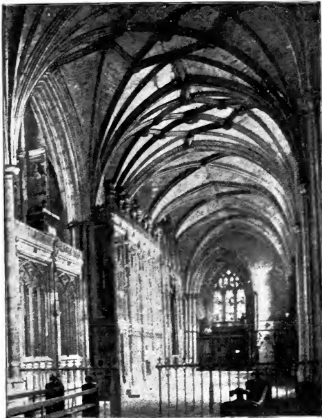
FIG. 76.—SOUTH AISLE OF WINCHESTER CATHEDRAL, ENGLAND.
