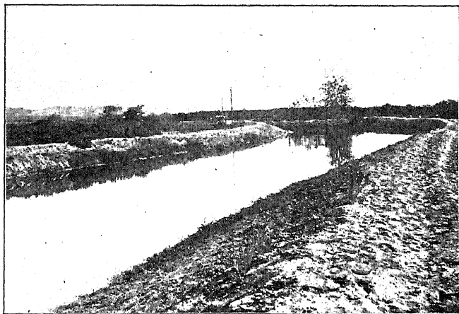
FIG. 52 b . Sunnyside Irrigation Canal, Washington
