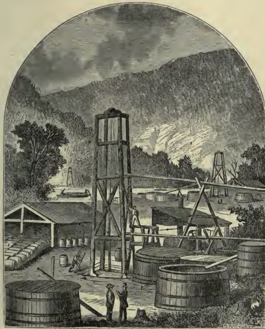
Fig. 138. Oil Well and Tank.
