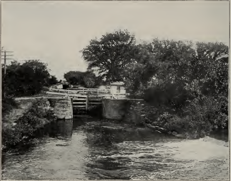
FIG. 67.—Locks at Channahon.
