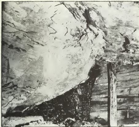
Figure 7 Channel cutting out the Herrin (No. 6) Coal at the abandoned Peabody Mine No. 9 in Christian County: view of the channel's edge, where the coal has been eroded at a 45° angle.
