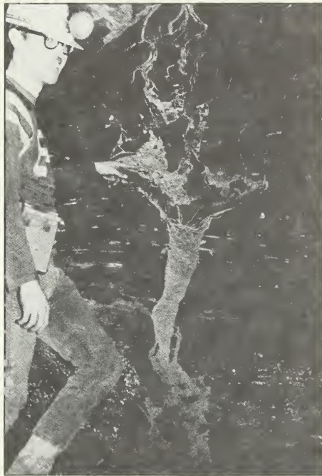
Figure 31 Clay dikes or horsebacks: (left) in the Springfield (No. 5) Coal at a surface mine in west-central Illinois; (right) in the Springfield Coal and overlying black shale at the abandoned El-Ben Mine in Logan County. The dike at the El-Ben Mine branches upward into myriad, small fissures, and veinlets that severely inhibit roof stability (photo shows Ronald Kern, formerly of the ISGS). (Photos by H. H. Damberger.)
