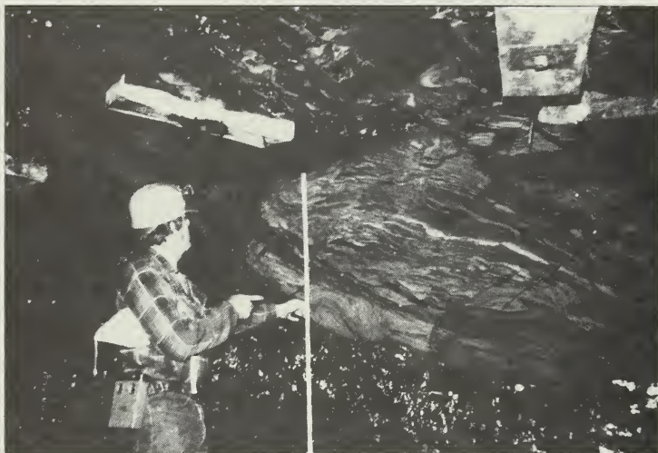
Figure 24a Part of a large sandstone-filled roll in the Herrin (No. 6) Coal at Inland Steel Mine No. 1 in Jefferson County. The lower part of the coal seam pitches sharply downward beneath the roll. (Chris Watson of Inland Steel Company is holding the ruler.)
