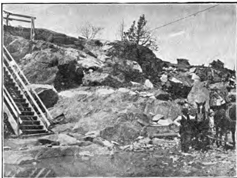
Fig. 2.—Riverside Drive and 93d St., north side, in process of removal, showing granite vein crossing quartzose gneiss.
