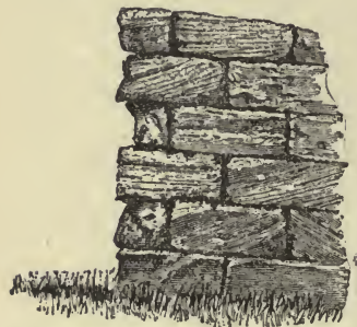
Fig. 1.— Weathering of rock, as shown by old masonry. (The “false-bedding” and other original structures of the stone are revealed by weathering.)
