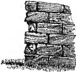
Fig. 1.—Weathering of rock, as shown by old masonry. (The “false-bedding” and other original structures of the stone are revealed by weathering.)
