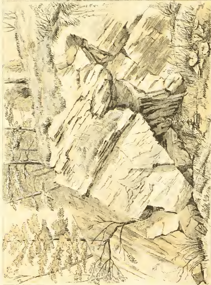
QUARRY AT WESTON, MASSACHUSETTS, SHOWING THE STRATA Showing absence of cleavage on N. side.
