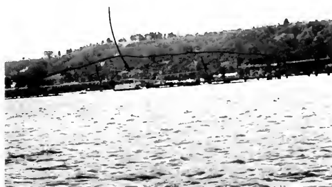
Photo 7. Fort Rosecrans landslide on Point Loma Peninsula, looking west. This slide mass is presently moving toward the east at a rate of approximately 10 centimeters per year.
