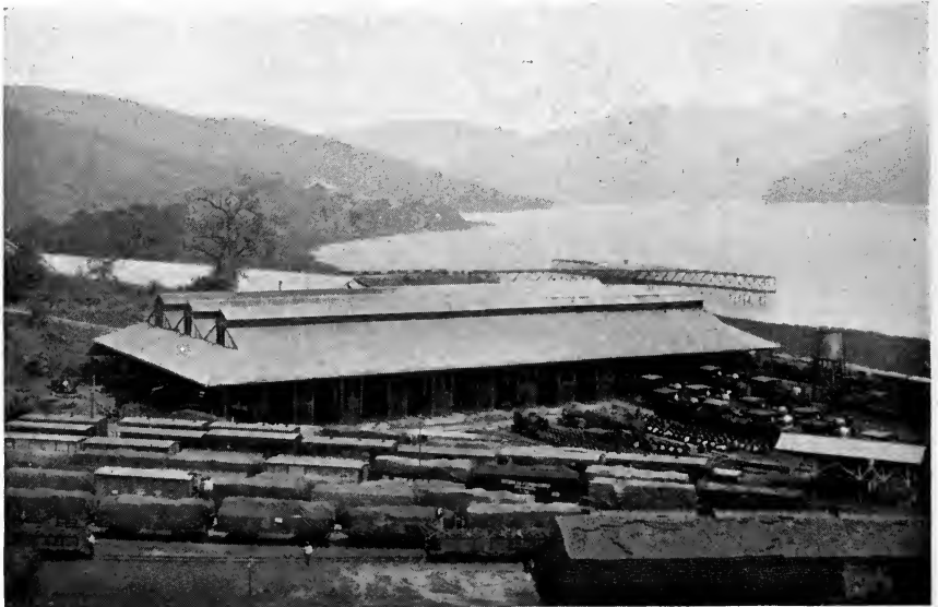
225. RAILWAY STATION, MATADI, LOOKING DOWN THE RIVER (On the promontory to the left are the buildings of the B.M.S. Base Station.)
