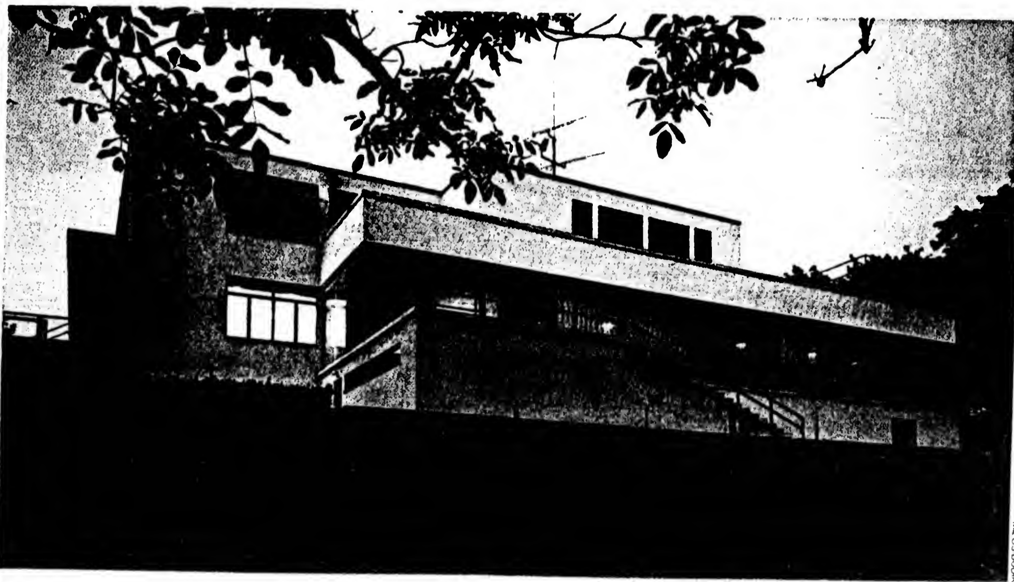
A view of the Tugendhat House at dusk displays the 15-foot-wide floor-to-ceiling windows of the 80-foot-long living space. Mies designed a system for raising and lowering the windows, which in the summer lent the main living space the feeling of a terrace.
