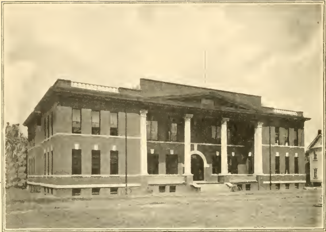
A Typical School Structure
