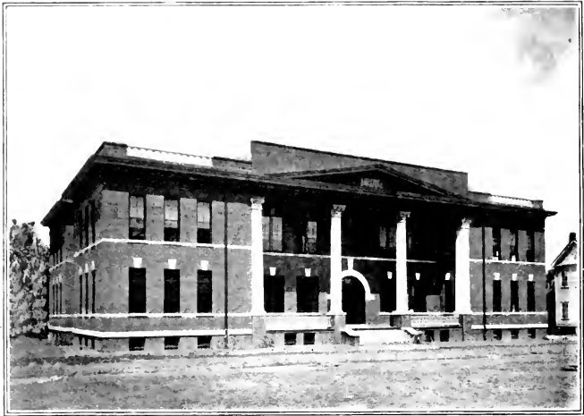
A Typical School Structure
