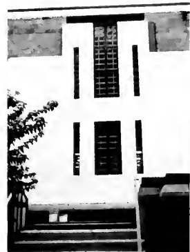
The wall after it was finished.
