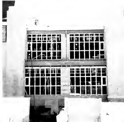
Near completion, the school begins to take form.
