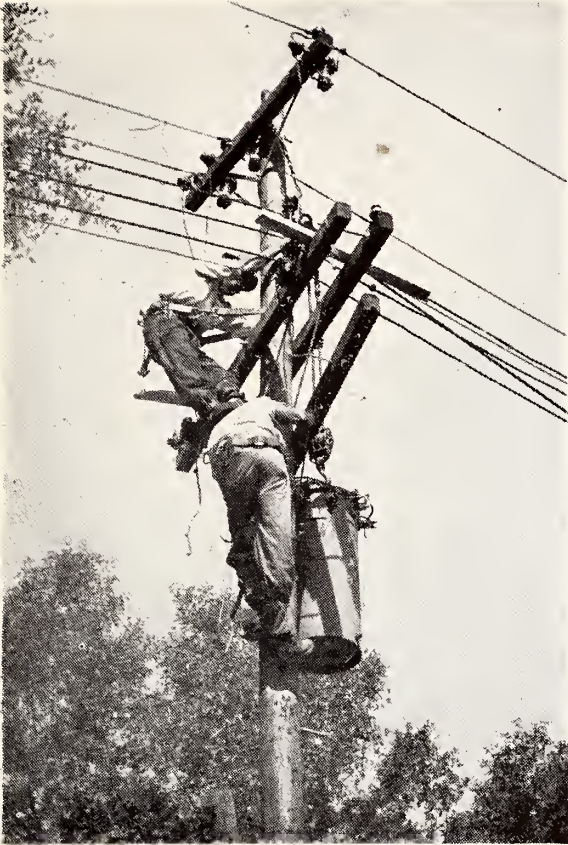
GEORGIA STATE COLLEGE STUDENTS OF ELECTRICITY: Doing Line Work
