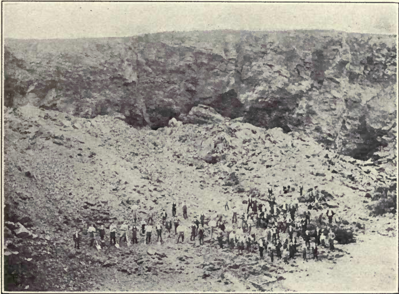
Fig. 2.—Gallery-work after the Blast.
