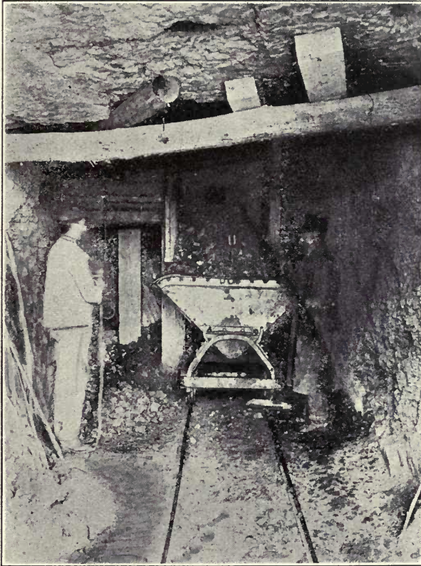
Fig. 4.—Car being Filled from the Glory-hole through the Sliding Door.
