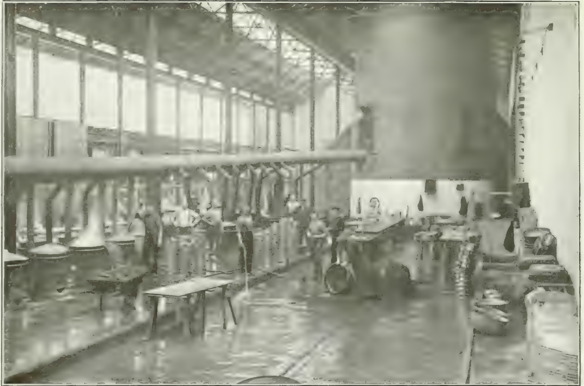
The Kitchens : Clearing Up.
