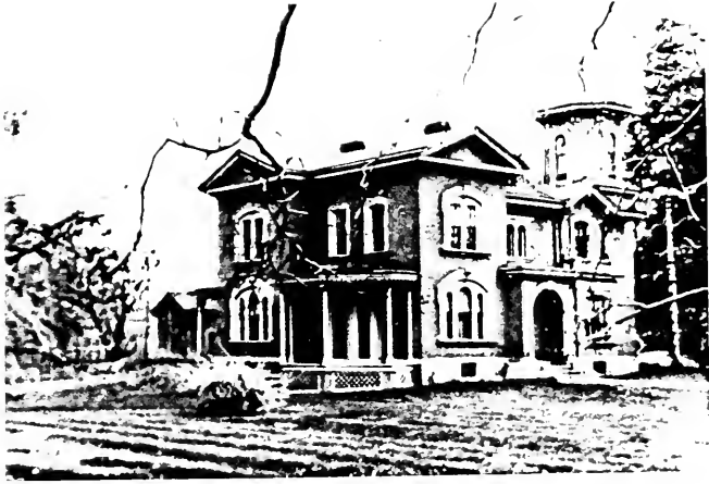
Wheeler: Patrick Barry House, Mount Hope Avenue, Rochester, New York, designed 1857 and constructed 1857-59.
