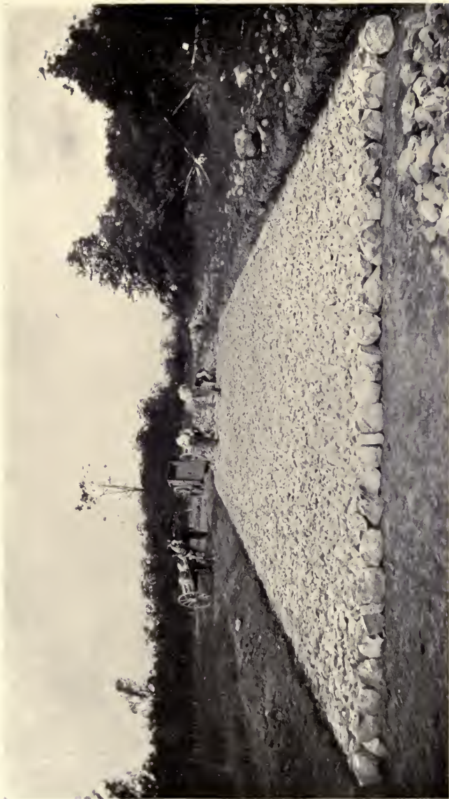
Cross-Section, Telford Avenue Foundation.
