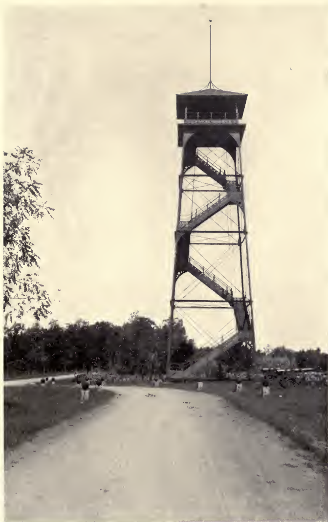
Tower on Confederate Avenue.
