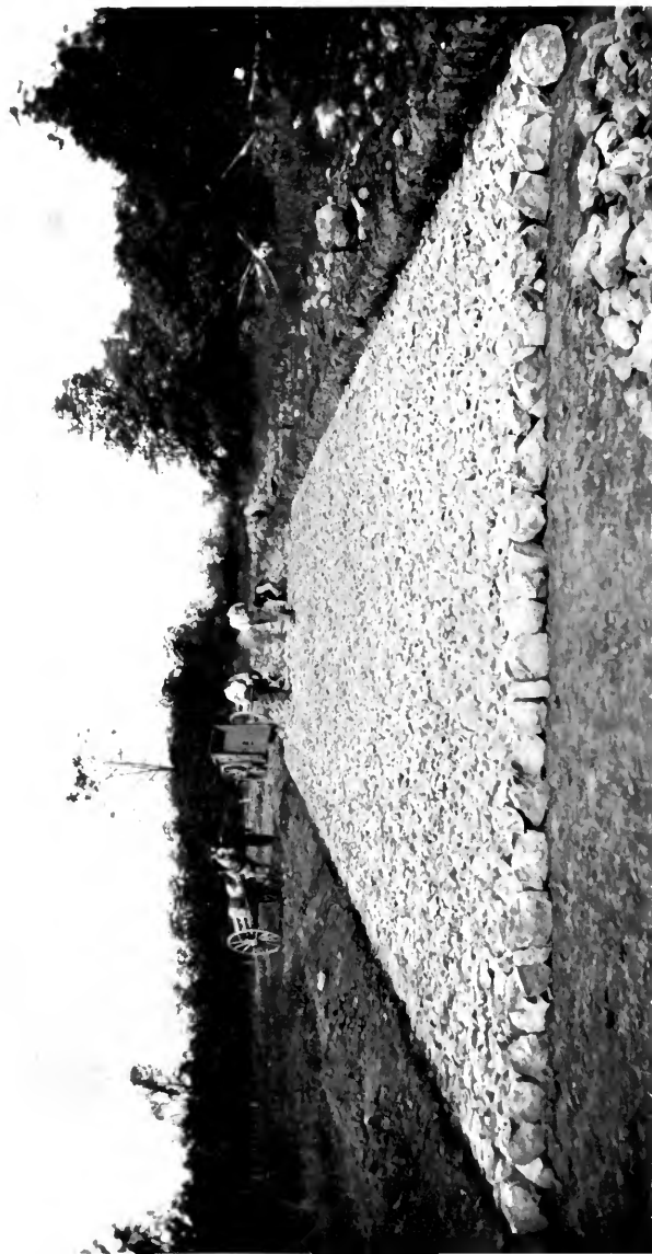
Cross-Section, Telford Avenue Foundation.
