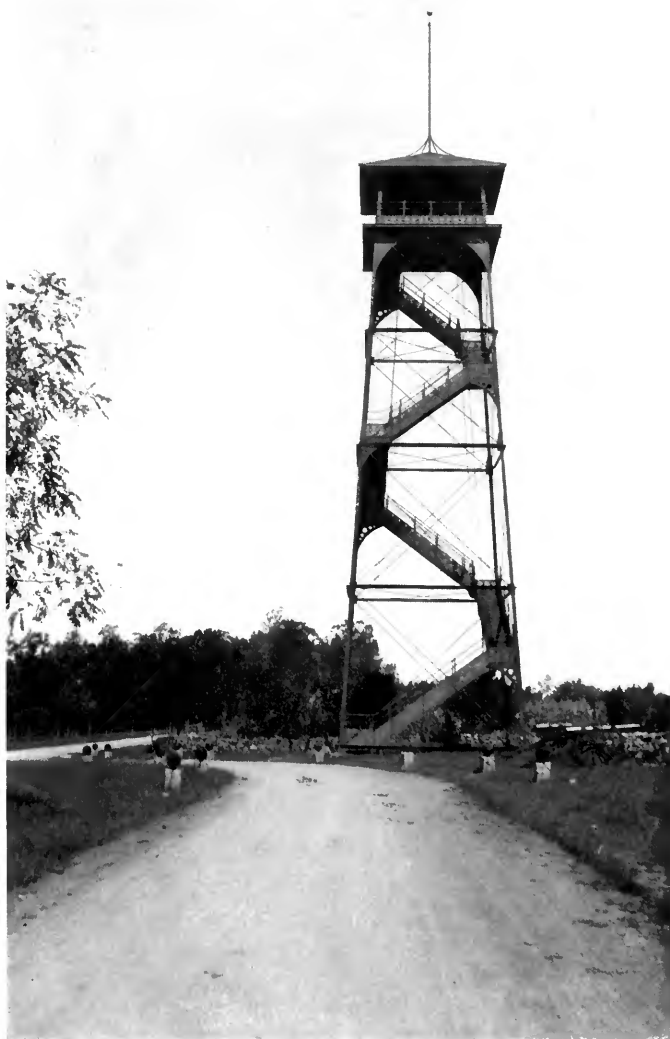
Tower on Confederate Avenue.
