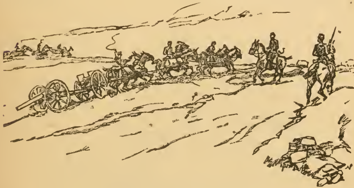
Getting the batteries into position.
