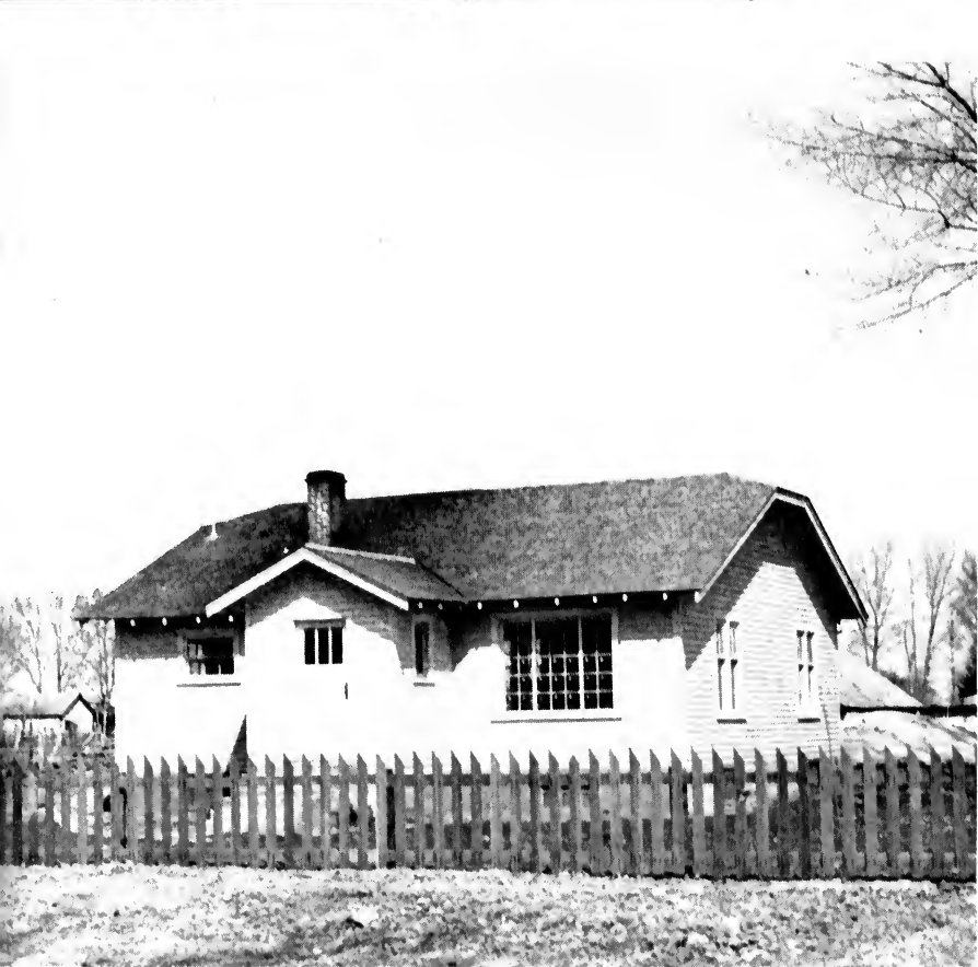
On the potato flats of Iona, Idaho, a family of eight lived in the one-room shack pictured at upper right. Another family of six occupied the shed shown at left. Organizing a self-help co-operative, the farmers built a new community. The lower photo shows a typical cottage in the development.
