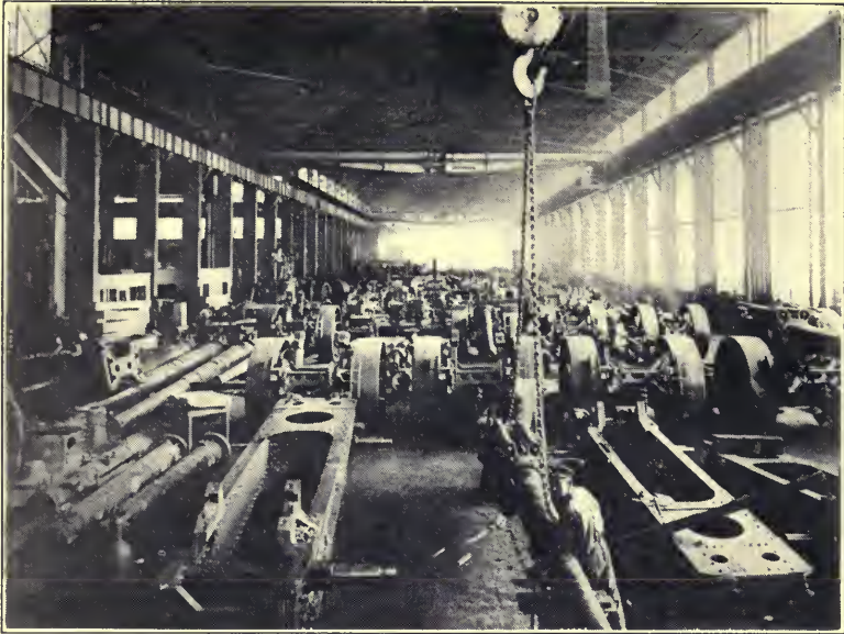
Photo from Morgan Engineering Company
