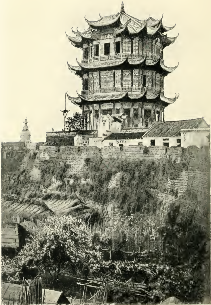
The Hua-Hua Lo at Wuchang, opposite Hankow ; one of the most beautiful pavilions in China, unfortunately destroyed by fire.
